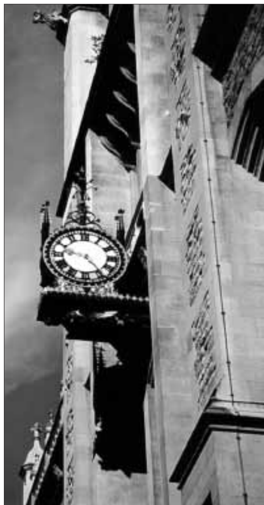
Clock tower that originally housed the water tank for the entire building and now contains study carrels
