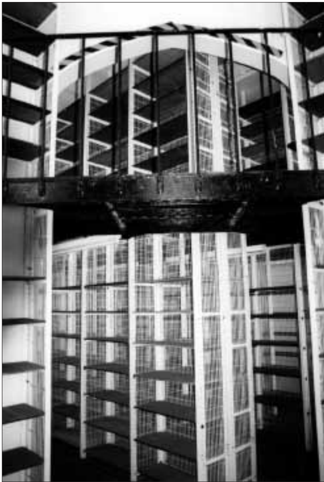
An original cell as used by PRO, the shelves being made of slate
