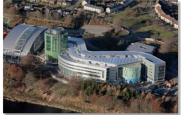
Photograph of phase 1 of the development from the riverside, November 2012
